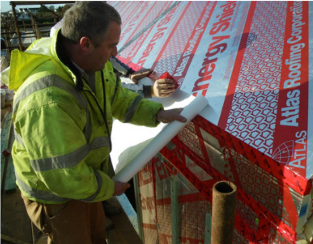
**Pictured is a textbook example of air tightness detailing. The crew is ensuring a continuous air barrier at the building's roofline.**
